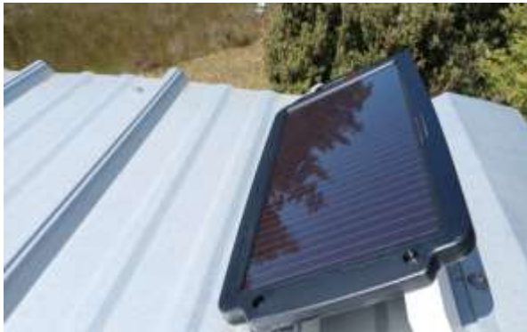
The solar panel is about 11" x 20" and we mounted it at an angle, facing southward, on the roof of the tiny house.
